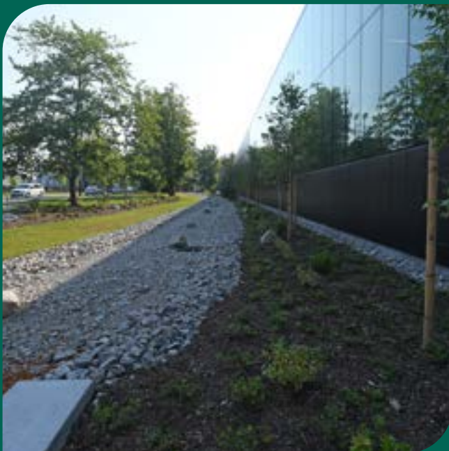
Vegetative bioswale outside of the Fitness Center.
