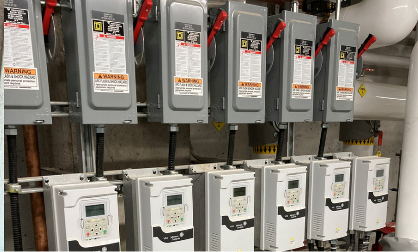
PHOTO 2.VARIABLE FREQUENCY DRIVES
