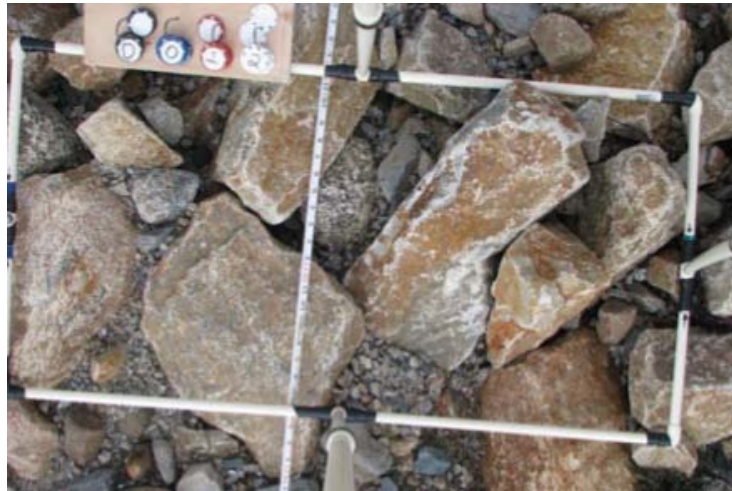
Figure 5. A photo showing the imported substrate (Thaumas Environmental Consultants Ltd., 2007).
