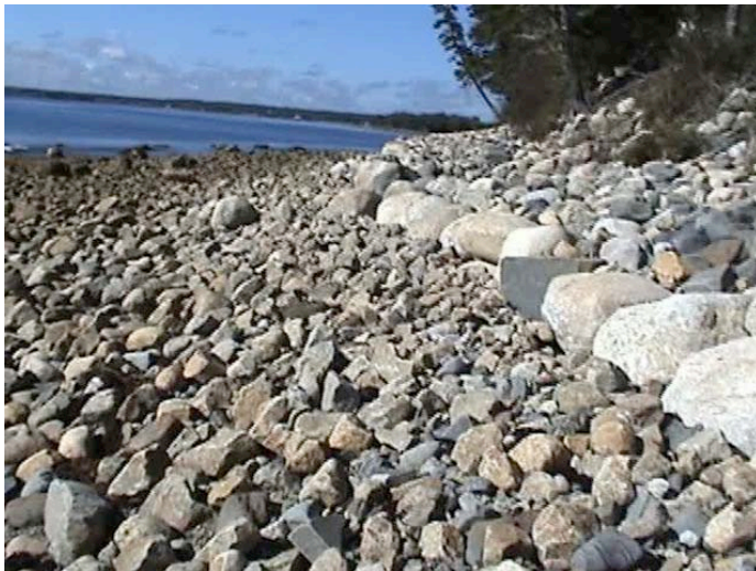
Figure 12. View of rock wall from line E looking towards line F.
